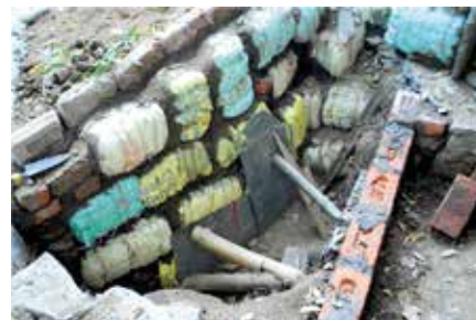
Walls filled with plastic waste constructed with plastic bricks/ plastic bricks walls a berm filled with non-biodegradable plastic.
