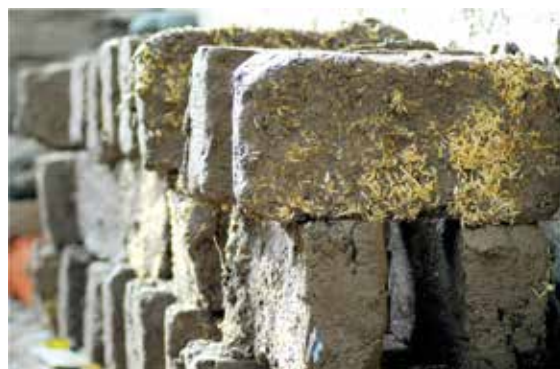
Brick with the rice husk to provide better binding and insulation: an incremental improvement in the excellent heat retention in Earthen building.
