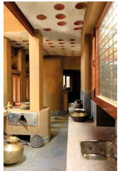
Improving the concept of wood burning smokeless chulha with an innovative design on a raised counter. Also, the use of a filler slab with local earthen pots to reduce the use of imported concrete.
