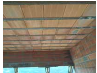
» Figure 5 Slab work with ISMB and Porothersm bricks
