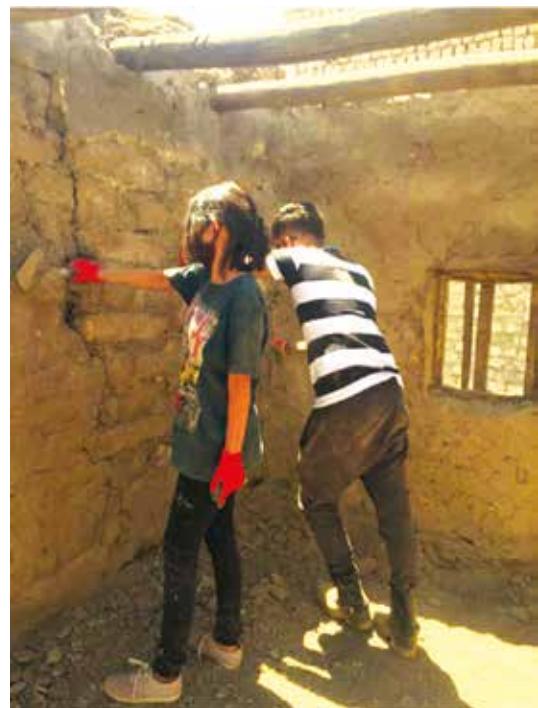
» Re-plastering the wall
