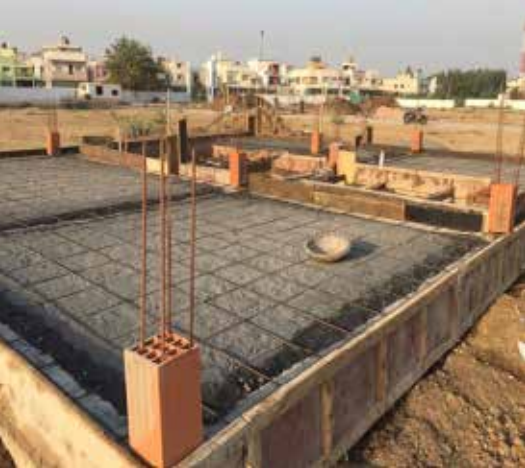
» Figure 1 Foundation work of APNA GHAR construction system
