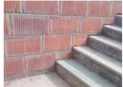
» Figure 4 Staircase made up of kadappa stones
