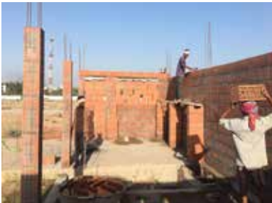
» Figure 2 Brickwork and columns of APNA GHAR construction system
