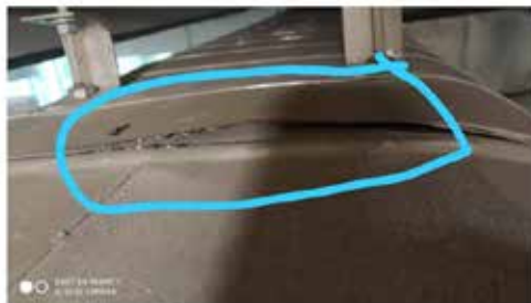
Duct Leakages at Sites
