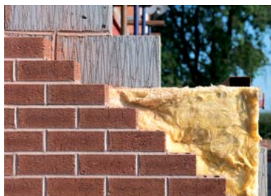
Photograph 4: Double brick-wall cavity insulation
