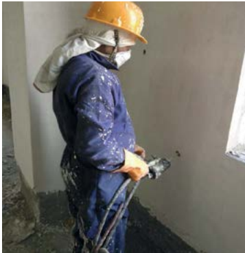
Photograph 8 (a): External-wall insulation with polyurethane chemicals poured in situ
