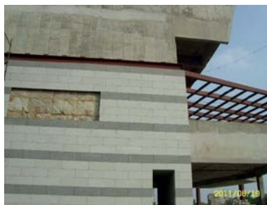
Photograph 5: Cavity wall insulation with aluminium stone finish
