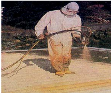
Photograph 3: Roof overdeck insulation with PUF slab and spray system
