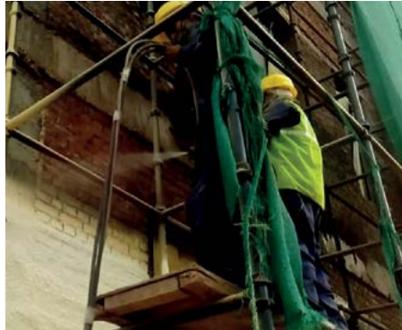
Photograph 8 (b): External-wall insulation with spray foam insulation
