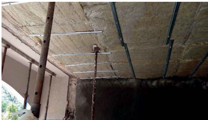
Photograph 1: Underdeck reinforced cement concrete insulation
