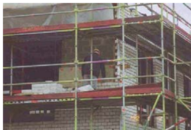
Photograph 6: Double brick-wall insulation
