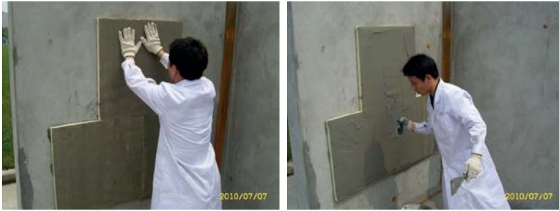
Photograph 7: External wall insulation with close cell CFC-HCFC free-rigid foam-slab insulation
