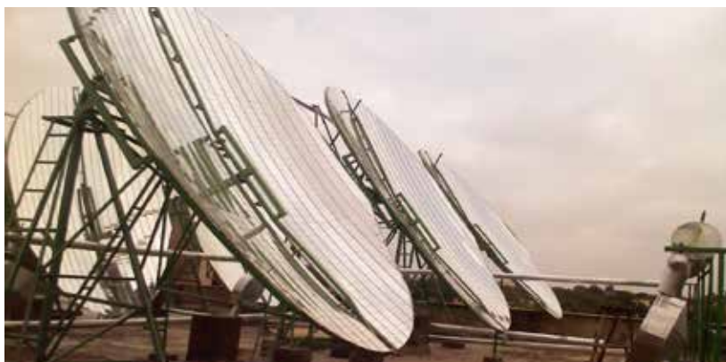
Picture 2: Solar Air Conditioning System Using Vapour-absorption Technology and Parabolic Concentrators.
