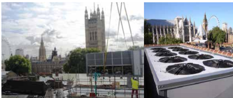
Picture 1: - R290 Chiller Installed at Church House, Westminster Abbey
